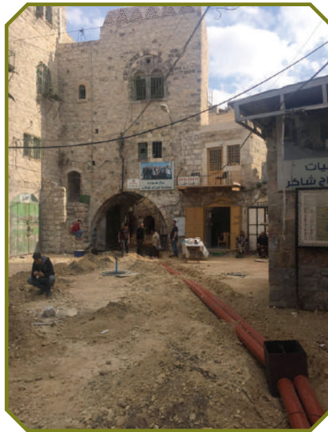
INSTALLATION OF PLASTIC PIPES FOR ELECTRICITY AND COMMUNICATION NETWORKS
