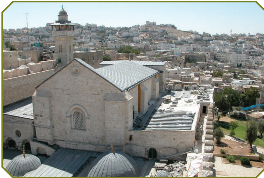
ROOF MAINTENANCE WORK
