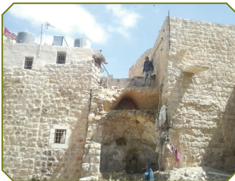
PART OF THE RESTORATION WORK IN THE AREA
