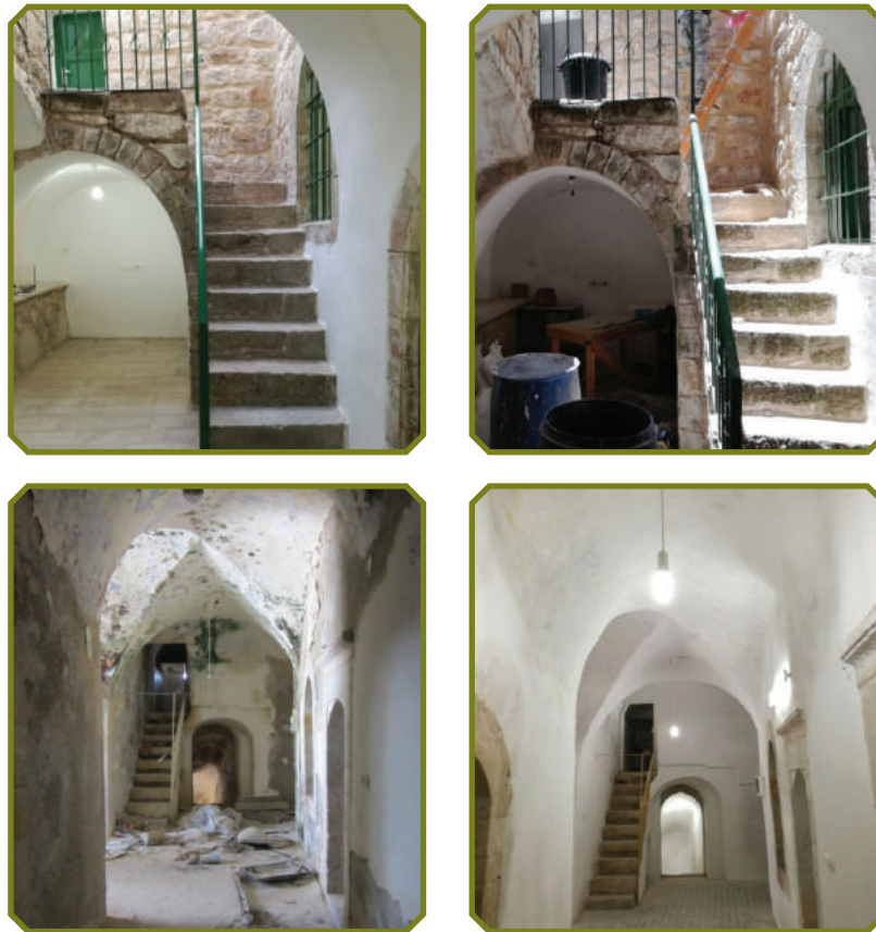
PICTURES SHOWING BEFORE AND AFTER MAINTENANCE WORK
