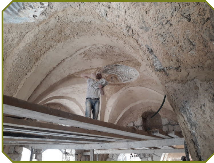
A VIEW OF THE EXECUTION OF THE WORK IN THE BUILDING
