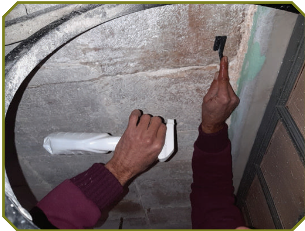
CLEANING STONES OF THE IBRAHIMI MOSQUE'S WALLS
