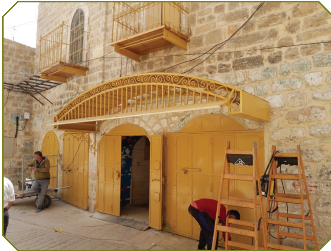
INSTALLATION WORKS FOR ONE OF THE SHOPS
