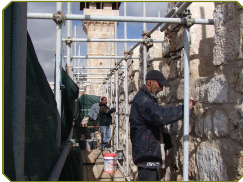
POINTING WORK ON THE EXTERNAL WALLS OF THE IBRAHIMI MOSQUE'S
