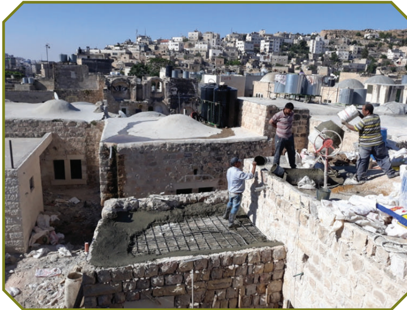
VIEW OF THE SURFACE INSULATION WORKS
