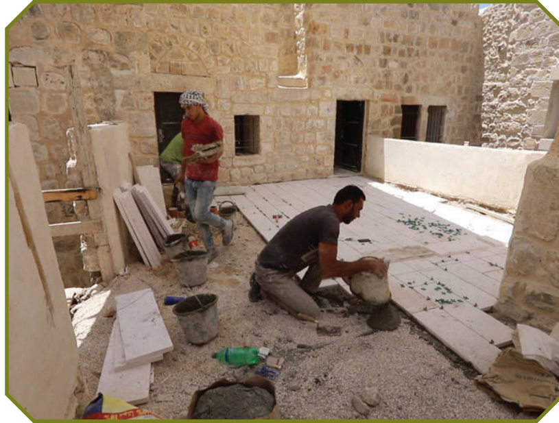
VIEW OF THE EXECUTION OF THE TILES
