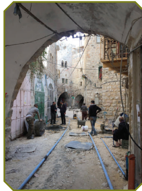
INSTALLATION OF PLASTIC PIPES FOR ELECTRICITY AND COMMUNICATION NETWORKS
