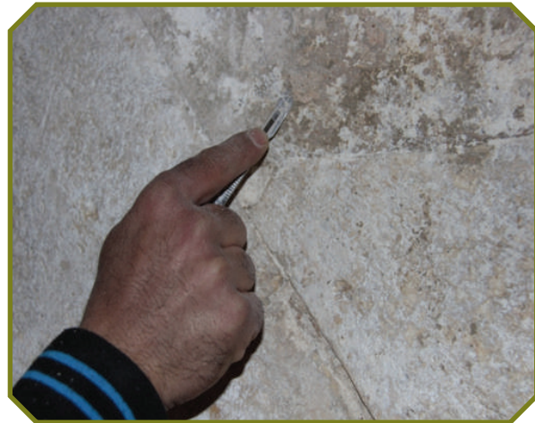
CLEANING STONES OF THE IBRAHIMI MOSQUE'S WALLS
