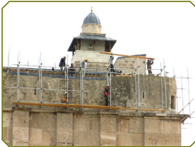
CLEANING THE UPPER PART OF THE EXTERNAL WALL OF THE MOSQUE
