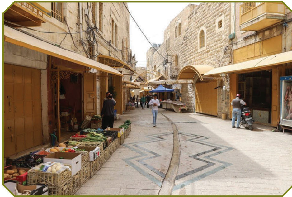
AL-QASABAH MARKET AFTER REHABILITATION
