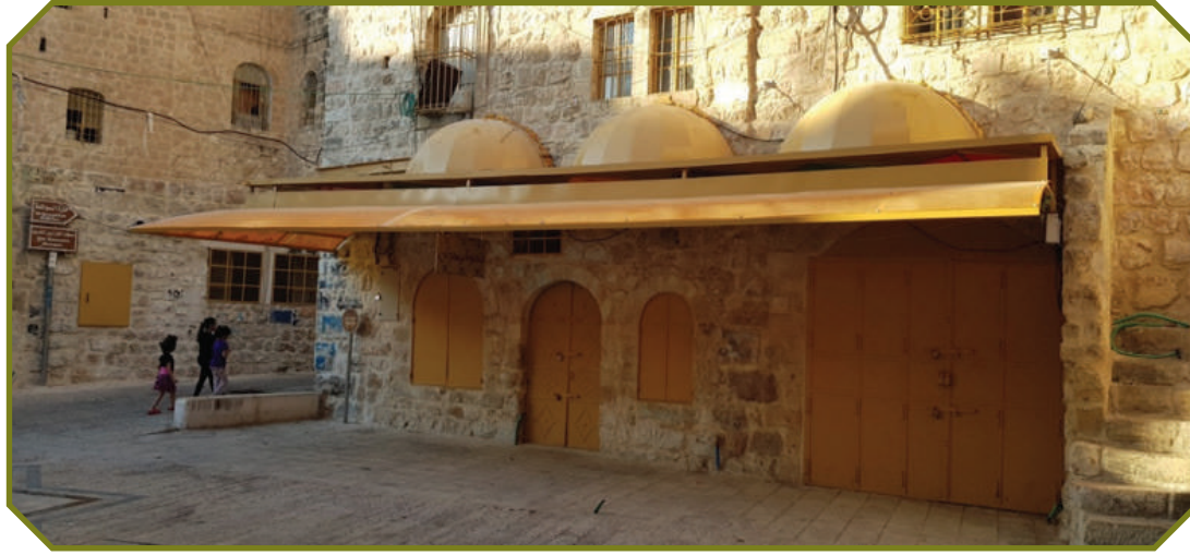
BADRAN CAFE UMBRELLA DURING INSTALLATION
