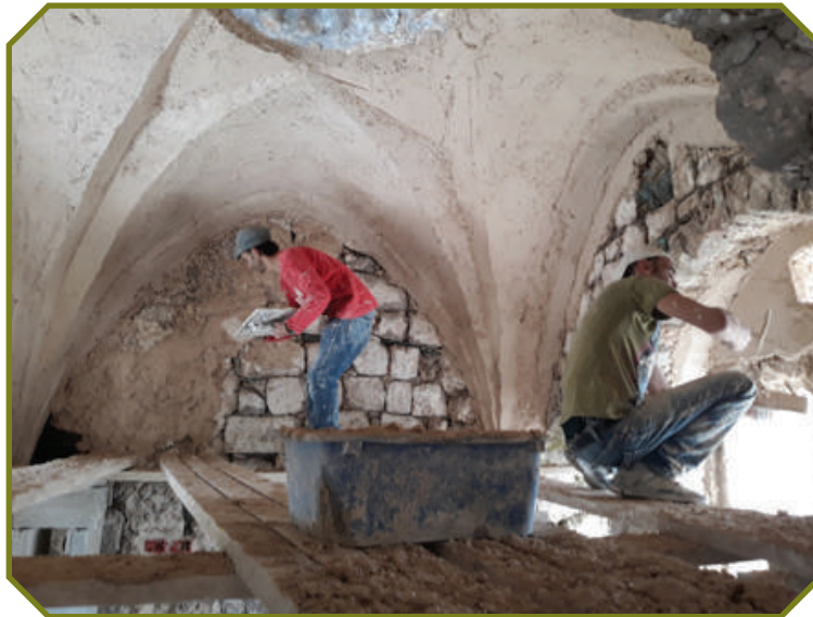
A VIEW OF THE EXECUTION OF THE WORKS OF INTERIOR LINING
