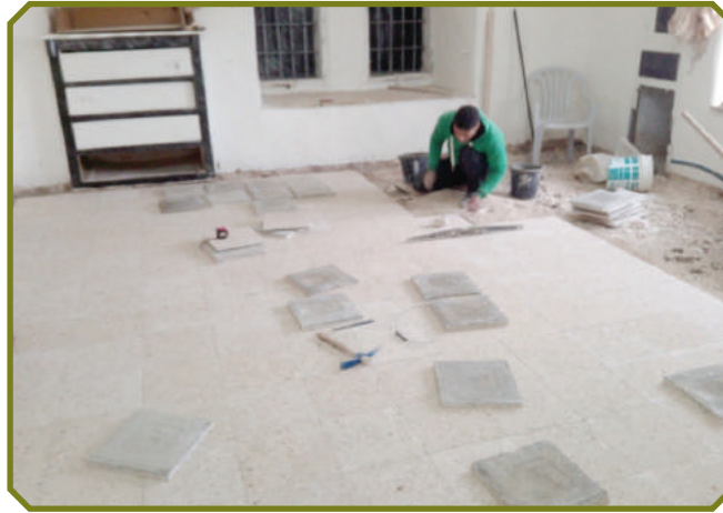
IMAGES SHOWING THE EXECUTION OF THE TILES DURING THE PROJECT
