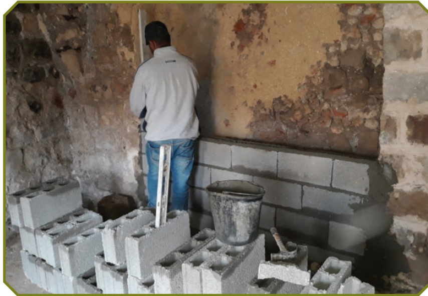
ELECTRICAL AND MECHANICAL WORKS
