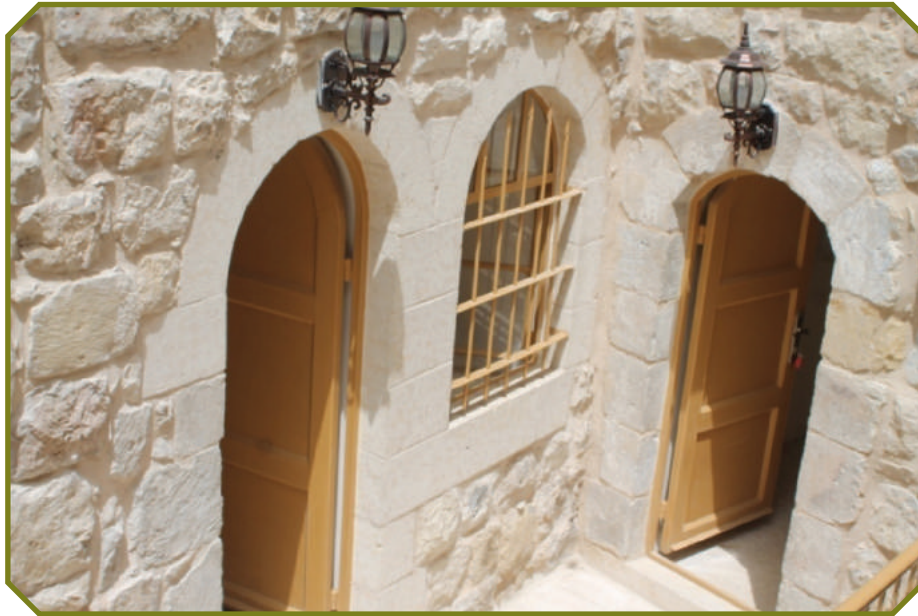
BEFORE AND AFTER RESTORATION
