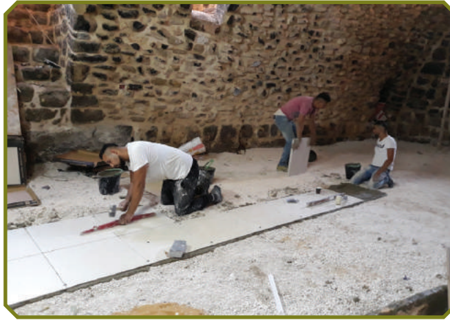
PLUMBING WORKS AND TILING FOR THE ENTRANCE OF THE SCHOOL
