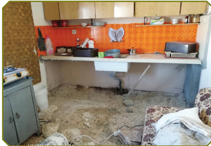
PART OF THE MAINTENANCE OF ONE OF THE BATHROOMS
