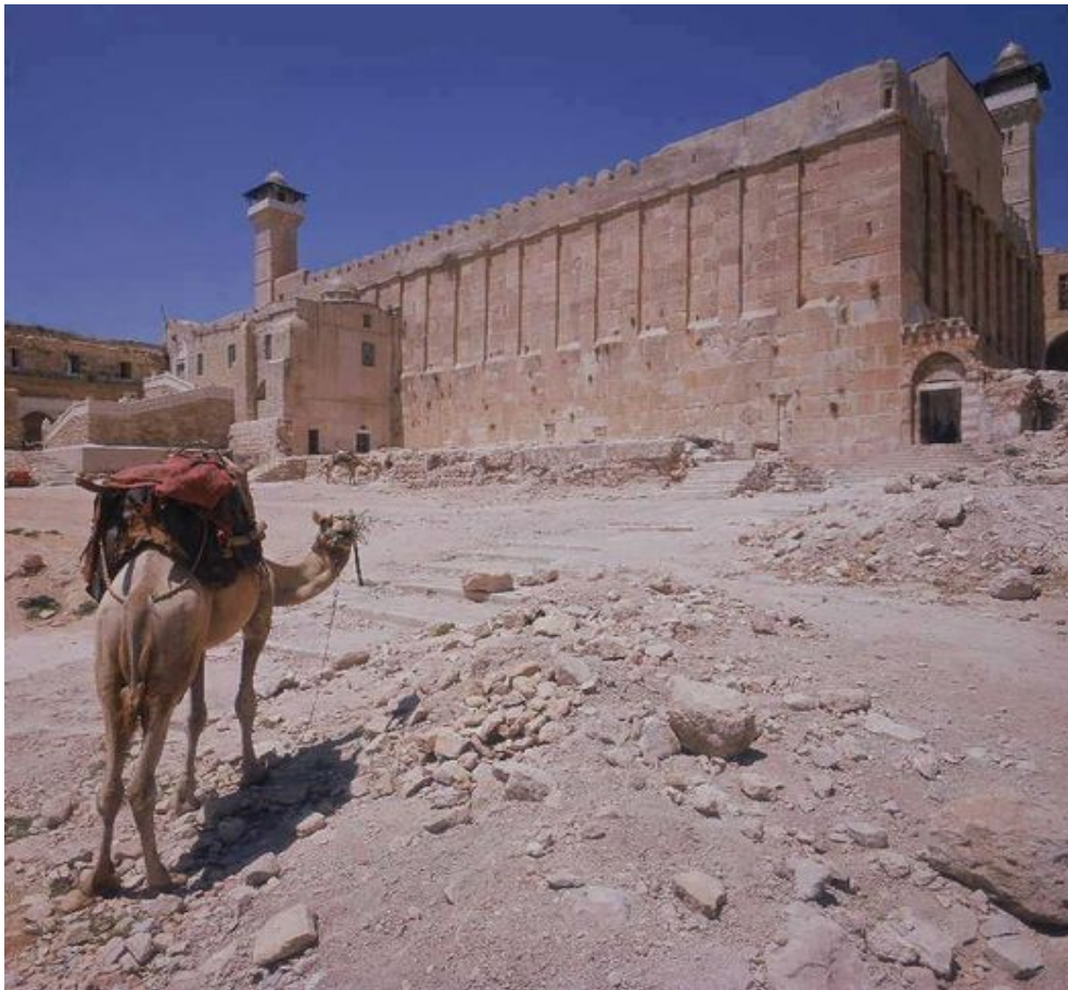
Photo taken after removing the buildings in front of the Ibrahimi Mosque
