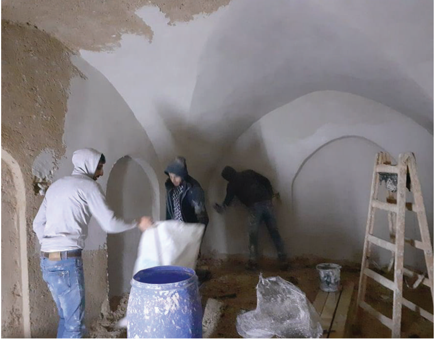
Before and After restoration
