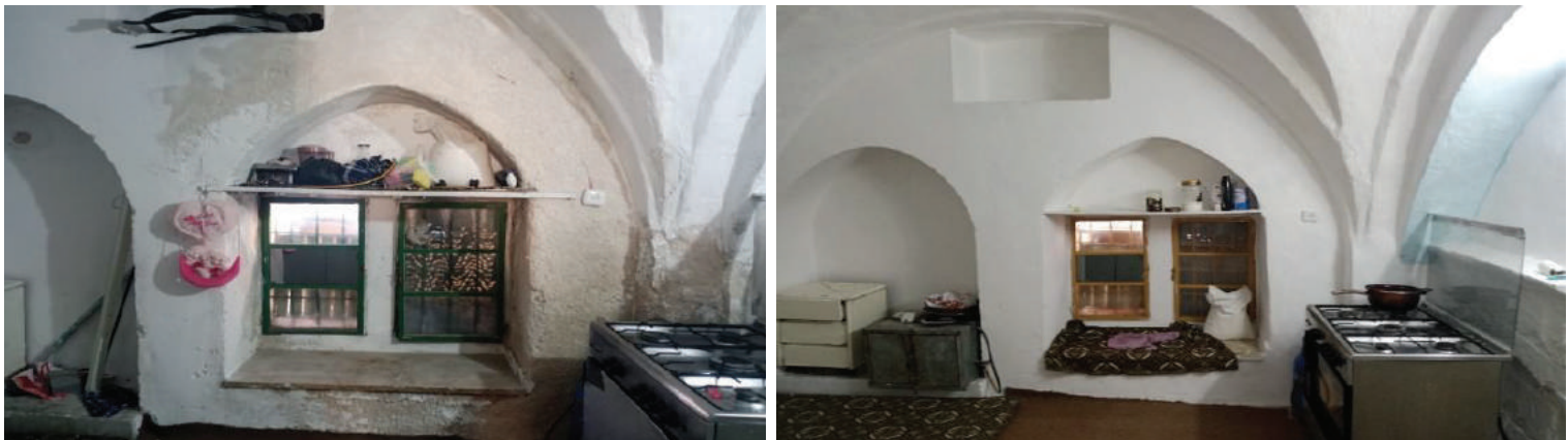
Before and After restoration
