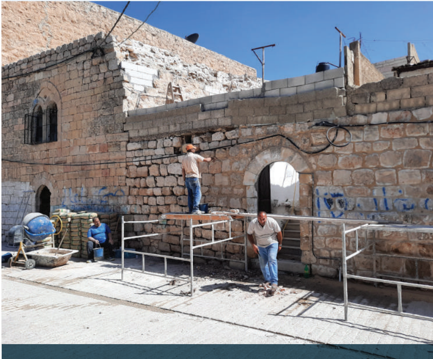
During restoration work
