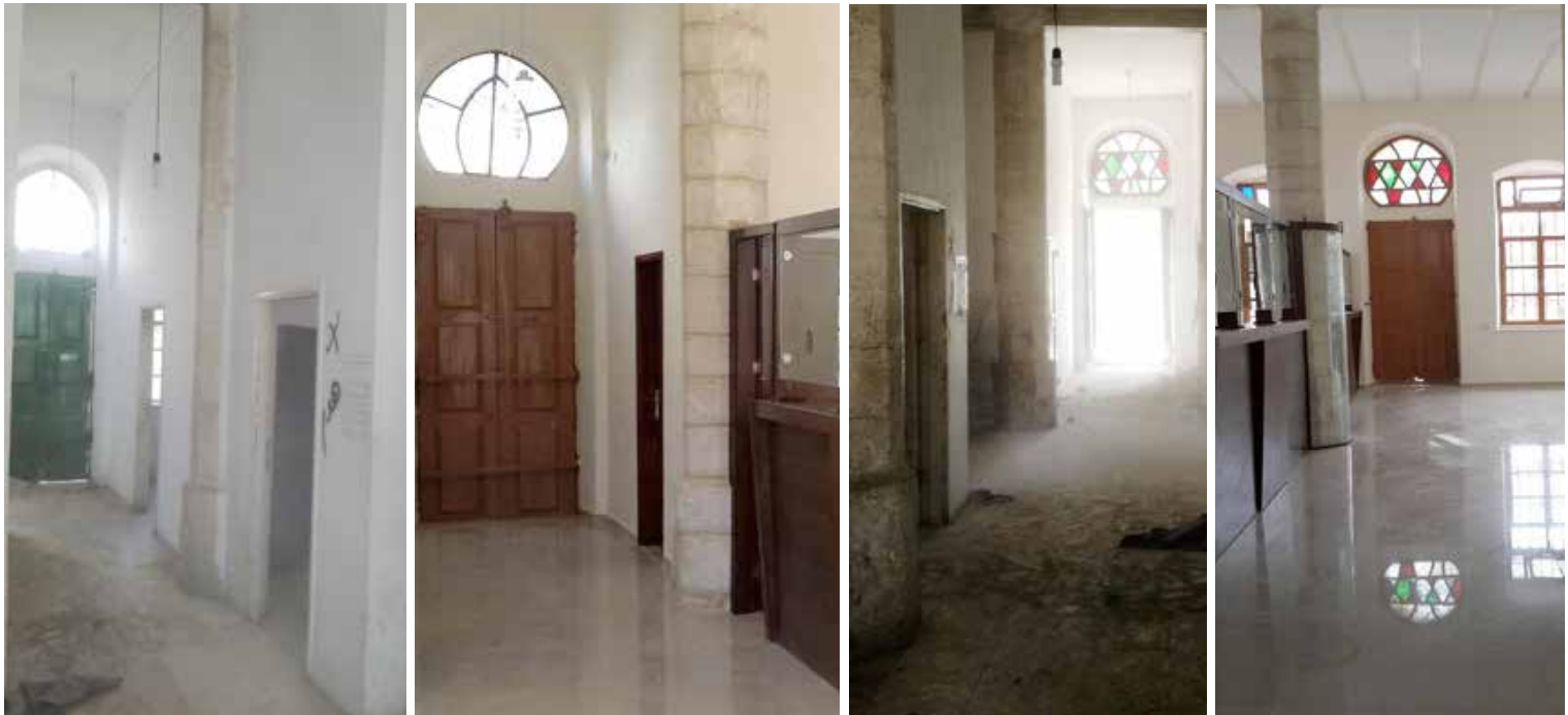
Before and after restoration
