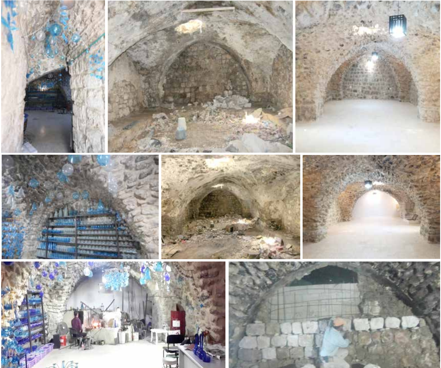
Before and after restoration of the Glass Factory hall
