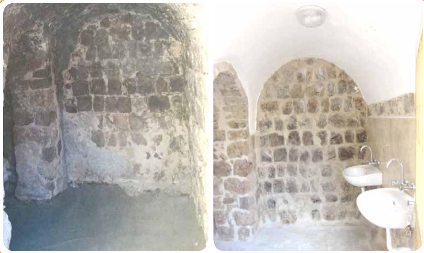
Before and after maintenance
