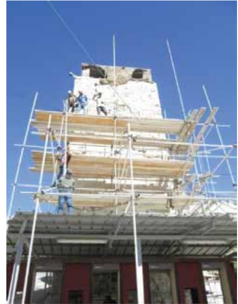
Tower Renovation Activities
