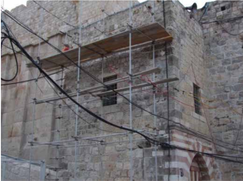
Renovating the Upper Room over the Western Entrance
