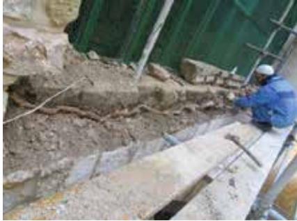
Renovating Eastern Entrance
