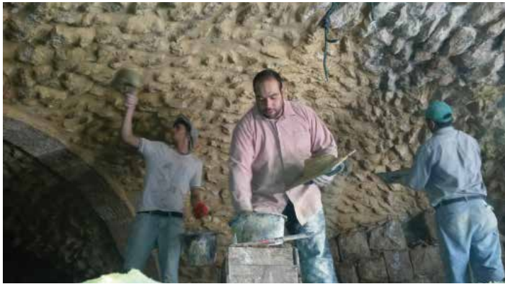
Photos taken during renovations
