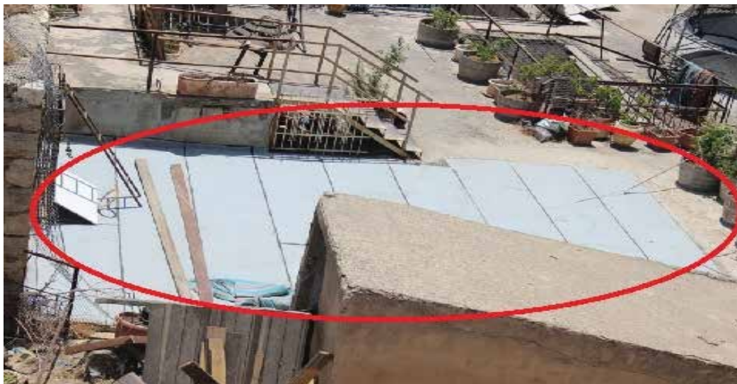
Photos of the roofs of Abu Munshar's stores after restoration
