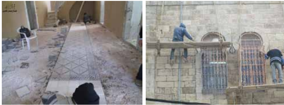
Part of schools renovation projects.
