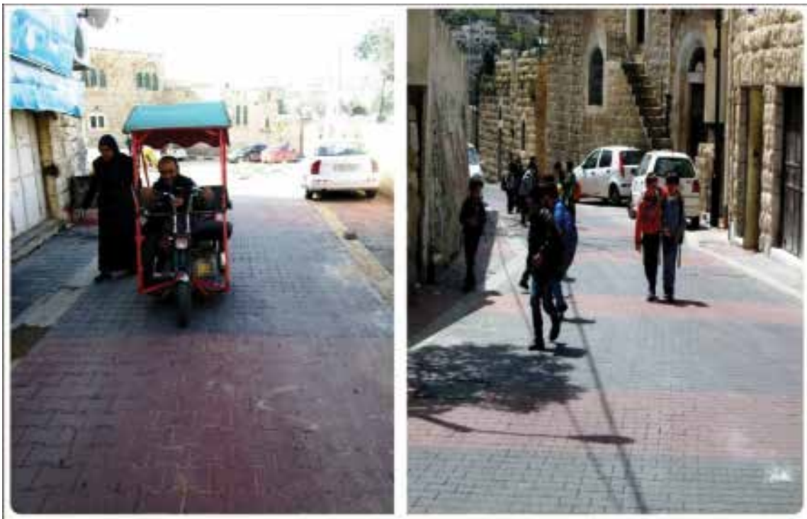
A photo of the area after infrastructure rehabilitation
