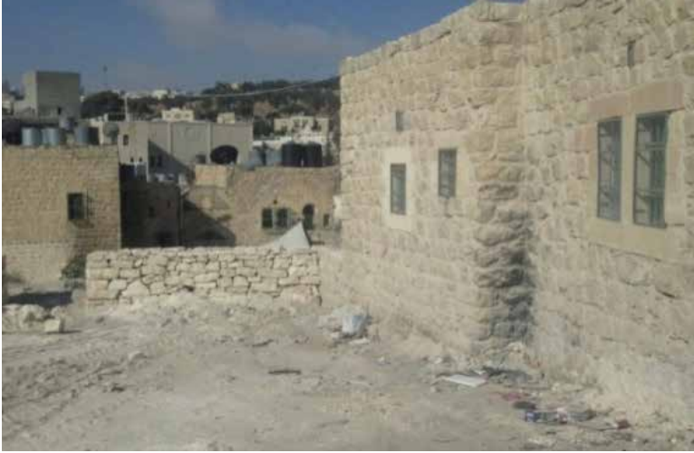
A photo of the yard before and during renovation
