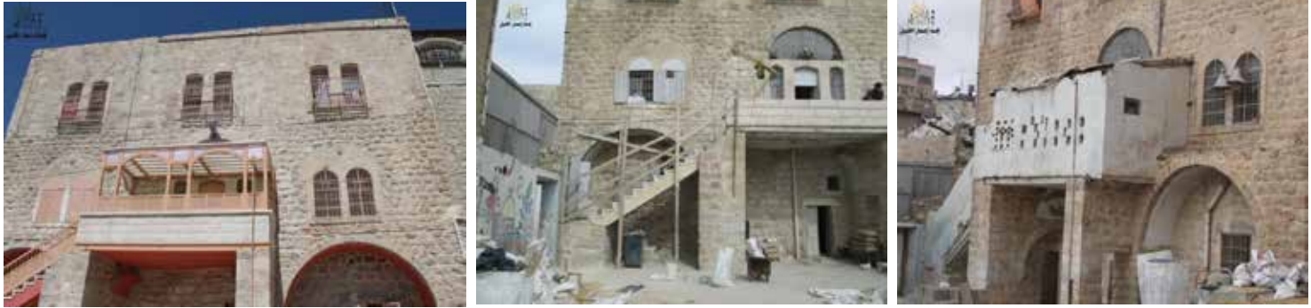
Main Facade of Yacobia School before and during renovation activity.
