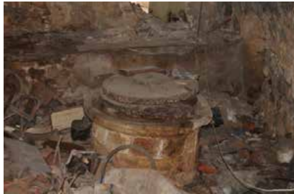
A photo of the press before renovation
