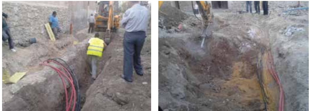
A photo of street during trenching works
