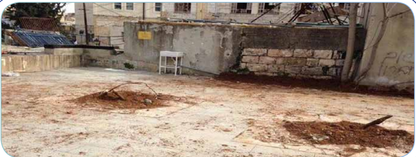
Image2: The floor of the station after removing the changes settlers placed on it.
