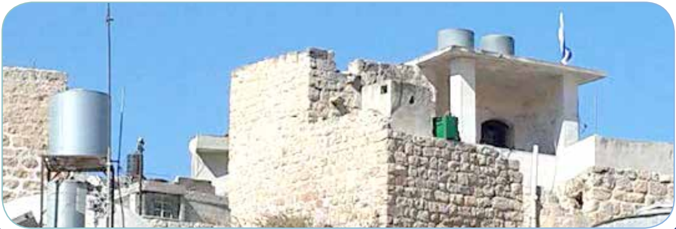
Image9: The old building inhabited by Yousef Rifai>ya, which was invaded by the occupation army
