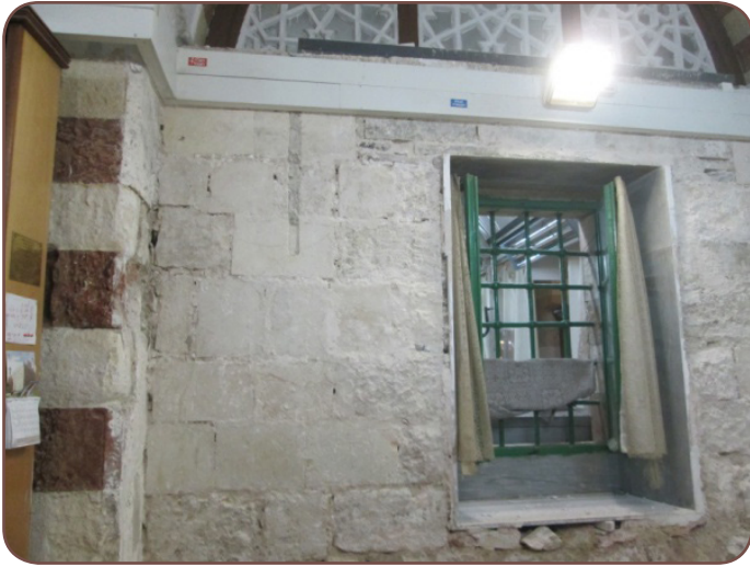
Carving the modern plaster (wall coating) and showing the original stone – Yusufia
