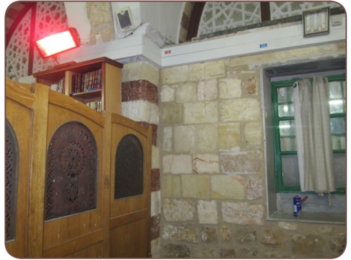
Carving the modern plaster (wall coating) and showing the original stone – Yusufia
