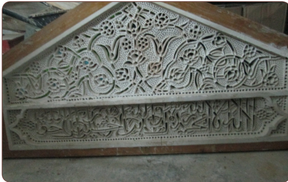
Maintenance of gypsum boards in El-Hadra El-Ibrahimia
