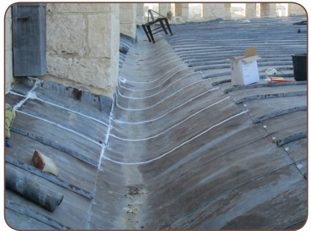
Maintenance of lead panels on roofs to prevent water leakage
