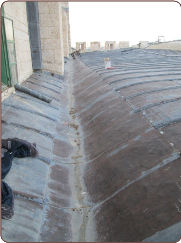
Maintenance of lead panels on roofs to prevent water leakage
